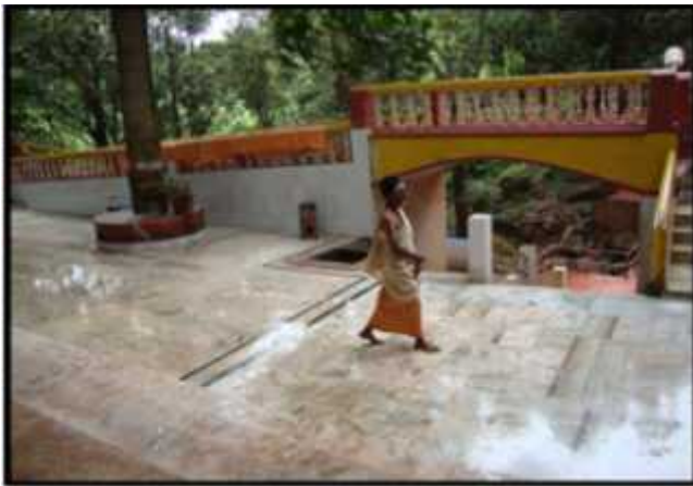
Photo -13A -Temple renovation work with Glazed Tile
