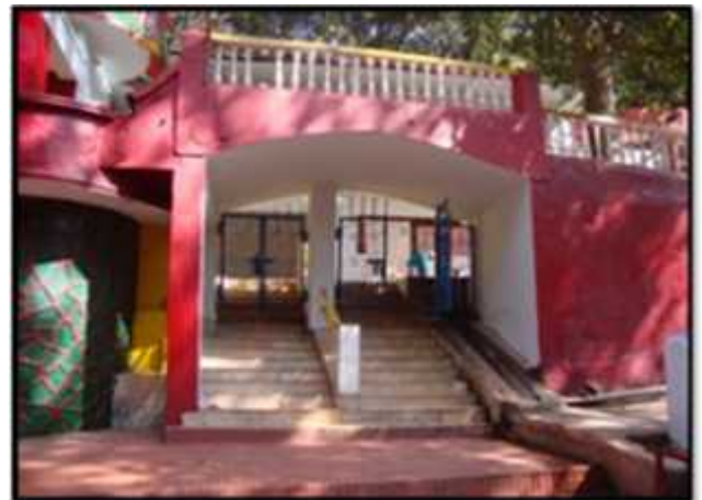
Photo -13B -Renovation work with Bench Tile & Coloring of walls
