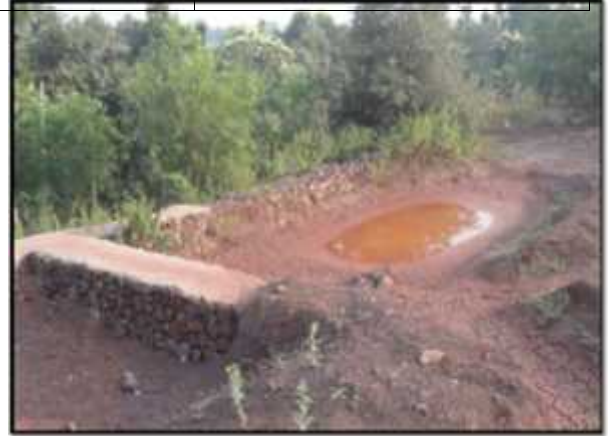
Photo 6 & 7– Settling cum harvesting Pit
