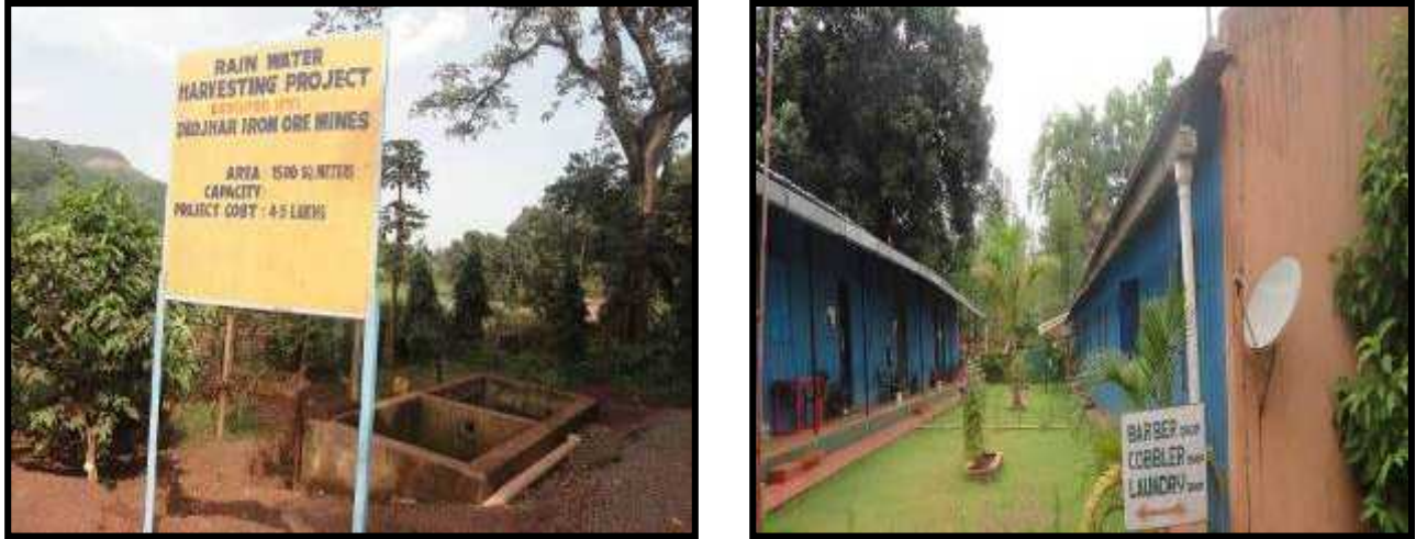
Photo 10 – Shows roof top Rain Water harvesting structure & Recharge Pit
